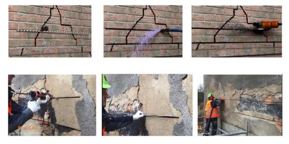
Figure 3. Increasing the shear and flexural strength of a brick wall with grouting (Afshari, 2017)
