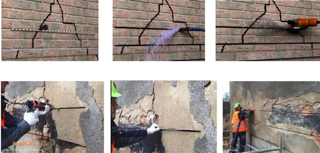
Figure 3. Increasing the shear and flexural strength of a brick wall with grouting (Afshari, 2017)
