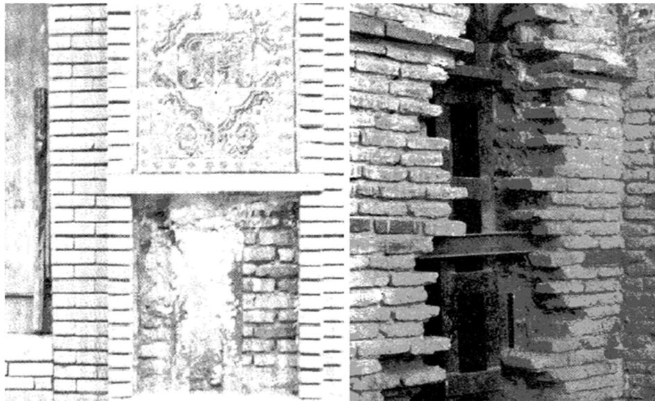
Figure 5. Embedding steel structural elements inside the wall "invisible form" (Mohebbali et al., 2014)
