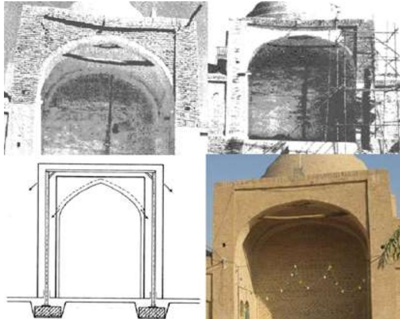
Figure 8. An example of the reinforcement of a portal with steel packing (Mohebbali et al., 2014)
