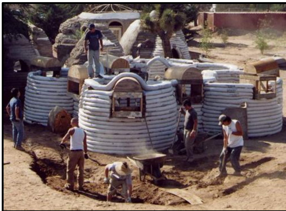
Figure 4. A sample of the sandbag house in California designed by Nader Khalili (Khalili, 2011).
