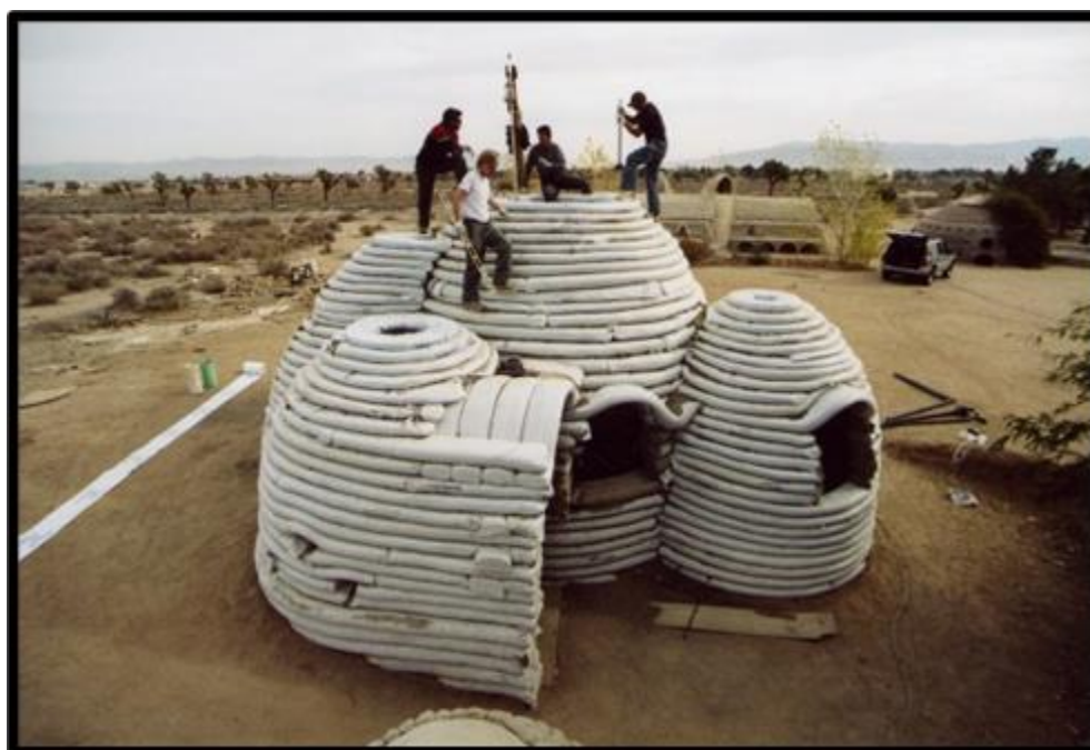
Figure 2. Sandbag house of Nader Khalili in Kuwait (Khalili, 2011).
