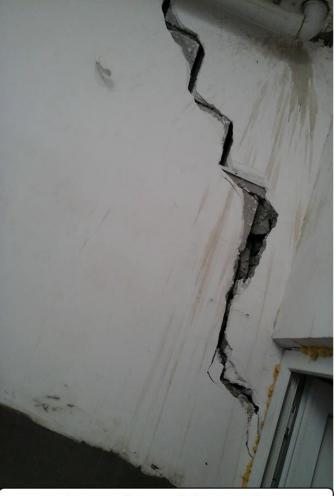
c. Diagonal stepped shear cracking
