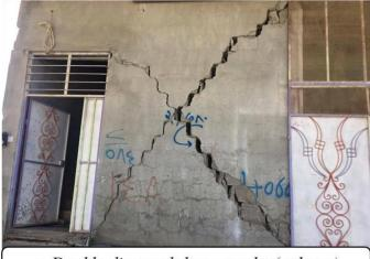
e. Double diagonal shear cracks (x shape)
