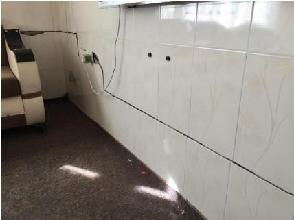
Figure 5. Horizontal Shear Crack at the Base of The Wall.
