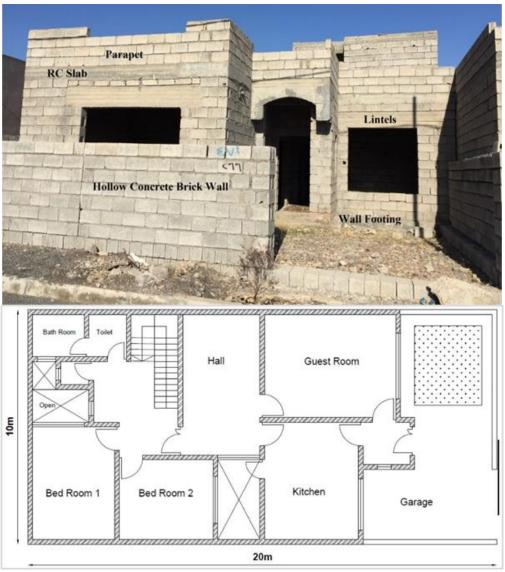
Figure 4. Typical Masonry House Components and Plan of a House.
