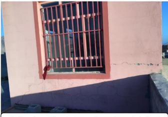
d. Cracks at the corners of openings (window)
