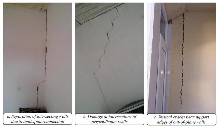
Figure 7. Corner Failure of Hollow-Block Masonry Houses.
