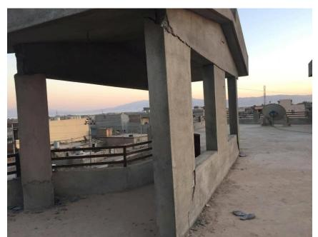
Figure 6. Cracks in Load-Bearing Masonry Walls With Many Openings.
