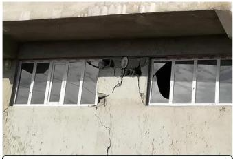
a. Cracking of spandrel wall between openings
