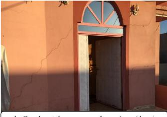
b. Cracks at the corners of openings (door)
