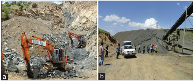
Figure 4. (a) Asnawa iron ore mine, (b) the crushing and sieving plant
