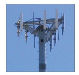
Figure 2. Top of a cellular radio tower. Nine sector antennae of three operators, three per one operator. http://en.wikipedia.org/wiki/Cellular\_ network
