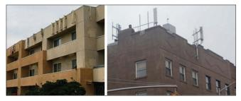
Figure 4. Photos show two examples of using cellular antennae that do not consider the safety guidelines (IEEE, 2006; FCC, 1997; ICNIRP, 1998) and distort the landscape.
