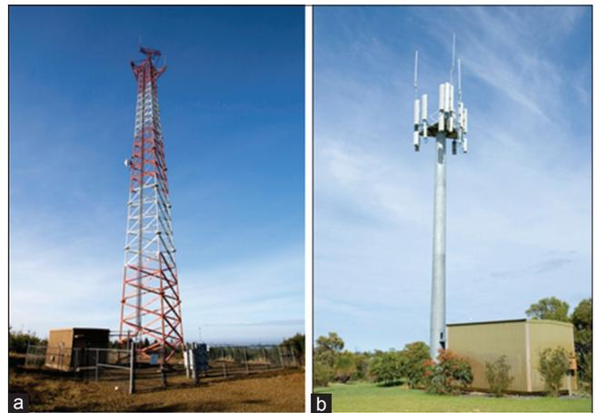
**Figure 1.** Photo of (a) latticework structure tower, and (b) monopole structure tower Photos are taken from: <http://www.fructivore.com/2010/10/look-for-the-right-short-candidates-like-crown-castle/>, [http://commons.wikimedia.org/wiki/File:Telstra\\_Mobile\\_Phone\\_Tower.jpg](http://commons.wikimedia.org/wiki/File:Telstra_Mobile_Phone_Tower.jpg).
