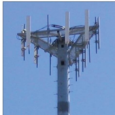
**Figure 2.** Top of a cellular radio tower. Nine sector antennae of three operators, three per one operator. [http://en.wikipedia.org/wiki/Cellular\\_network](http://en.wikipedia.org/wiki/Cellular_network)
